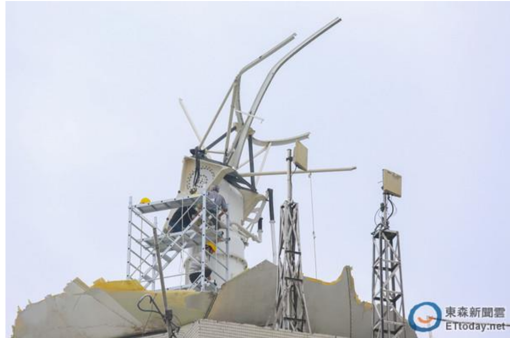
Wufenshan weather radar destroyed by Super Typhoon Soudelor (1513) Credit: Ettoday.net
