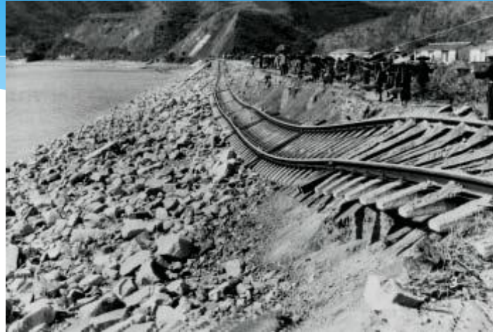
The railway track at Sha Tim damaged by a typhoon in 1937. (Courtesy Hong Kong SAR Public Records Office)
