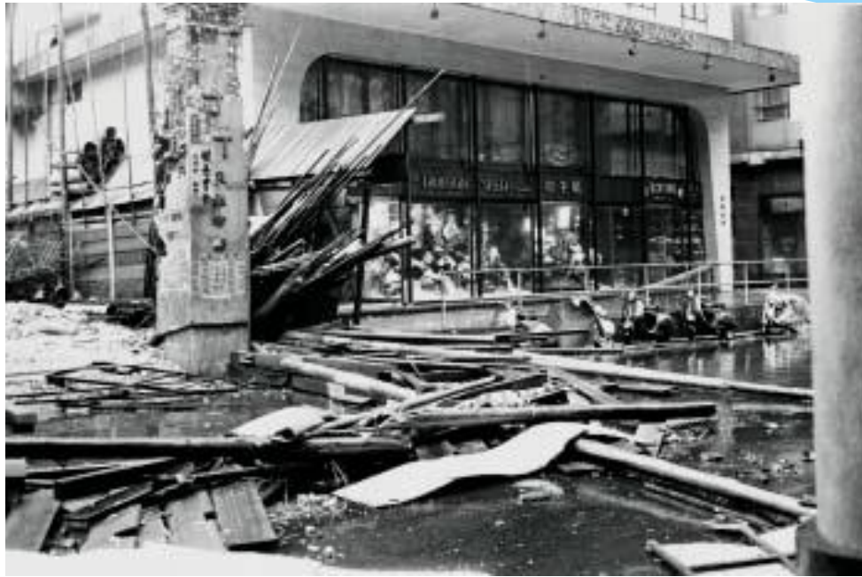
Damaged by typhoon Wanda . Courtesy Hong Kong SAR Information Services Department
