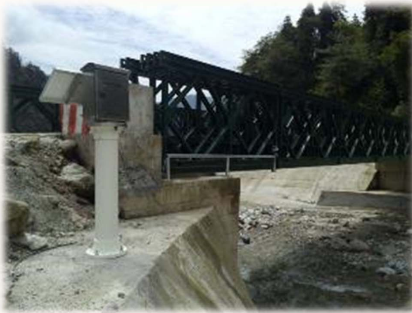
Water level gauge
