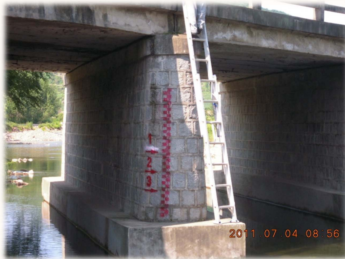
A simple gauging station at a bridge pier
