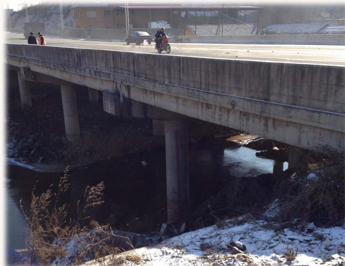
A simple water stage gauge at bridge pier
