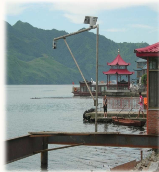
A radar water level gauge on-the-spot scene
