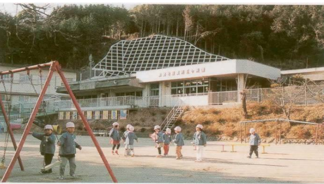
Protecting child welfare facilities with grating crib works
