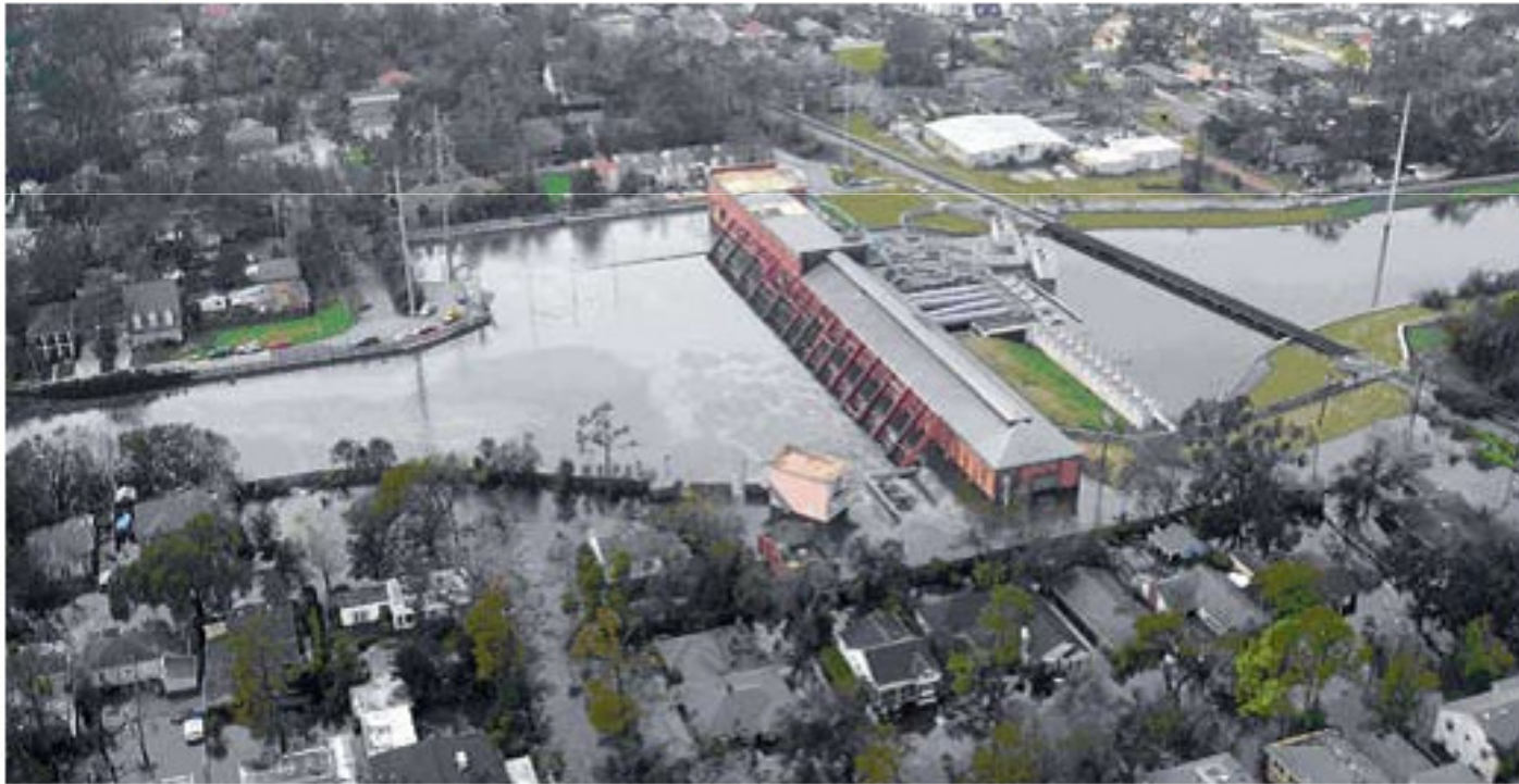
Rapid and far-reaching flooding caused by the hurricane protection system failure left most pump stations, such as Station No. 6 (on the 17th Street Canal), inoperable.
