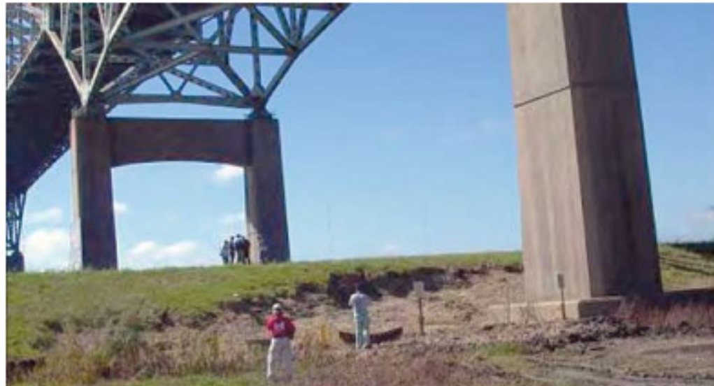
Levee Under the Paris Road Bridge in New Orleans East
