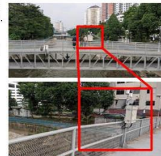
Installation of water level gauges on site.
