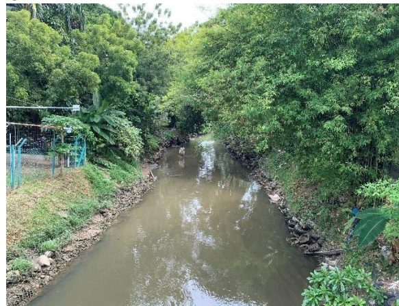
Figure 2-20 Sg. Pinang di Jalan P.Ramlee Water Level and Rainfall Observatory and Observation Section
