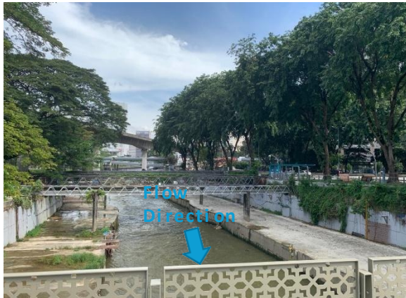
Figure 2-20 Sg. Kelang di Jam. Sulaiman Water Level Observatory Exterior
