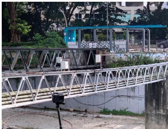
Figure 2-7 Sultan Sulaiman Bridge Water Level and Rainfall Observatory and Existing Water Level Gauge and Radio Velocity Gauge (non-contact type)
