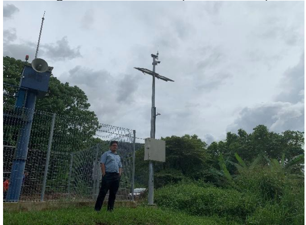
Figure 2-16 Web camera and siren device
