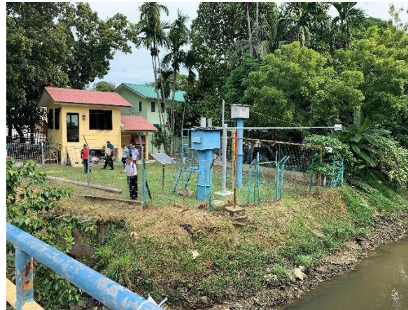
Figure 2-19 Sg. Pinang di Jalan P.Ramlee Water Level and Rainfall Observatory and Observation Section
