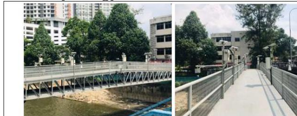
Figure 2-26. The summary of the installation date of WLG is shown in the Table 2-3 below.
