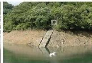
Reservoir monitoring system introduction site (in Kochi prefecture)
