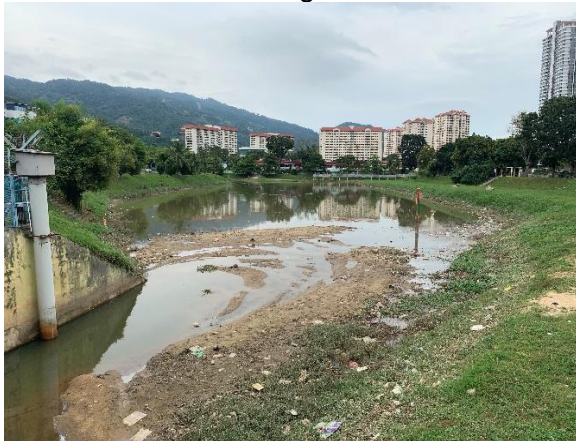
Figure 2-24(2) Kolam Sg. Dondang Water Level and Rainfall Observatory and Retarding Basin
