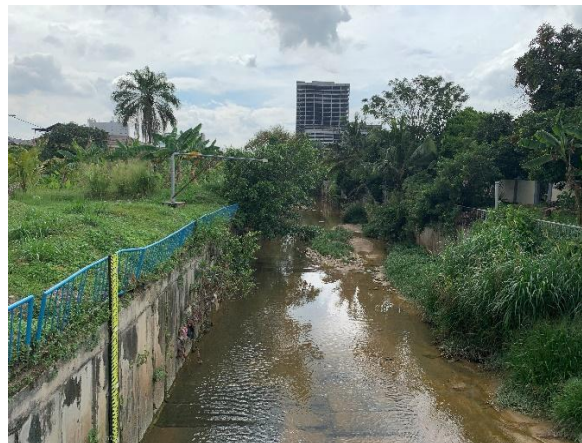
Figure 2-13 Kg. Sg. Kantan Water Level and Rainfall Observatory and Observation Section
