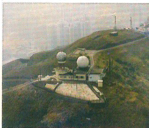
Tate's Cairn Radar Station overlooking Kowloon to the southwest. The Doppler Weather Radar (right) is shown with a protective radome alongside a Digital Weather Radar (left) installed in 1983. (Courtesy of Government Flying Services, Hong Kong)
