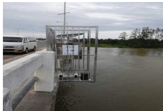
Water level gauge installed in 2013
