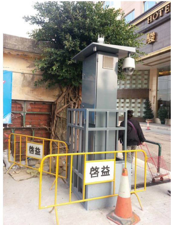
The new water level monitoring station
