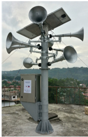
Warning post installed in 2014
