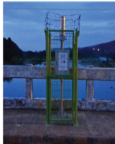
Rainfall gauge installed in 2014
