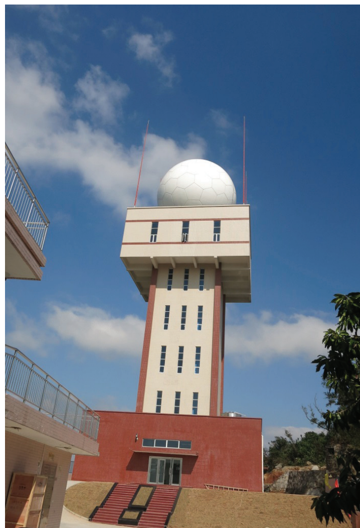
The new S band Dual-Polarization Doppler Weather Radar at Sanzhou town, Zhuhai
