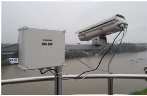
Intelligent CCTV overlooking the Cagayan De Oro River
