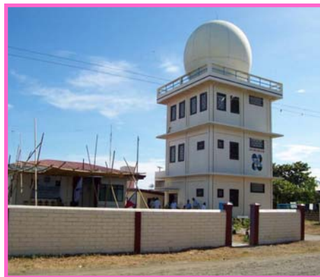
View of Aparri radar
