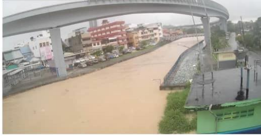
Kajang Water level Station before overflow
