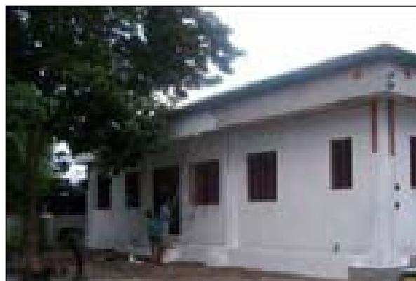
Figure 25. The new Pampanga River Flood Forecasting and Warning Center
